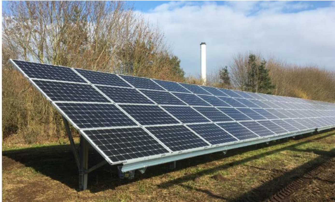
Figure 4: Example of a ground mounted solar PV array 4 - panel height at Briar Chemicals
